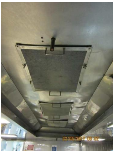
Exhaust trunking – CO2 nozzle inside
