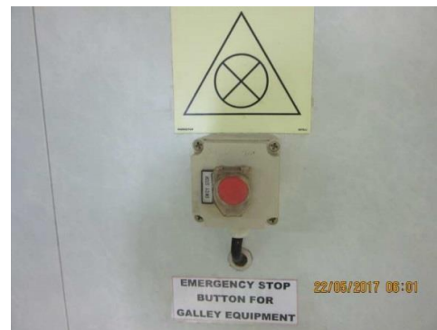
Emergency stop for galley fan outside galley
