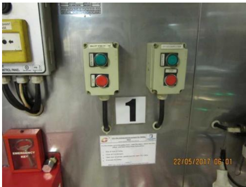
Galley exhaust and supply fan stops inside galley
